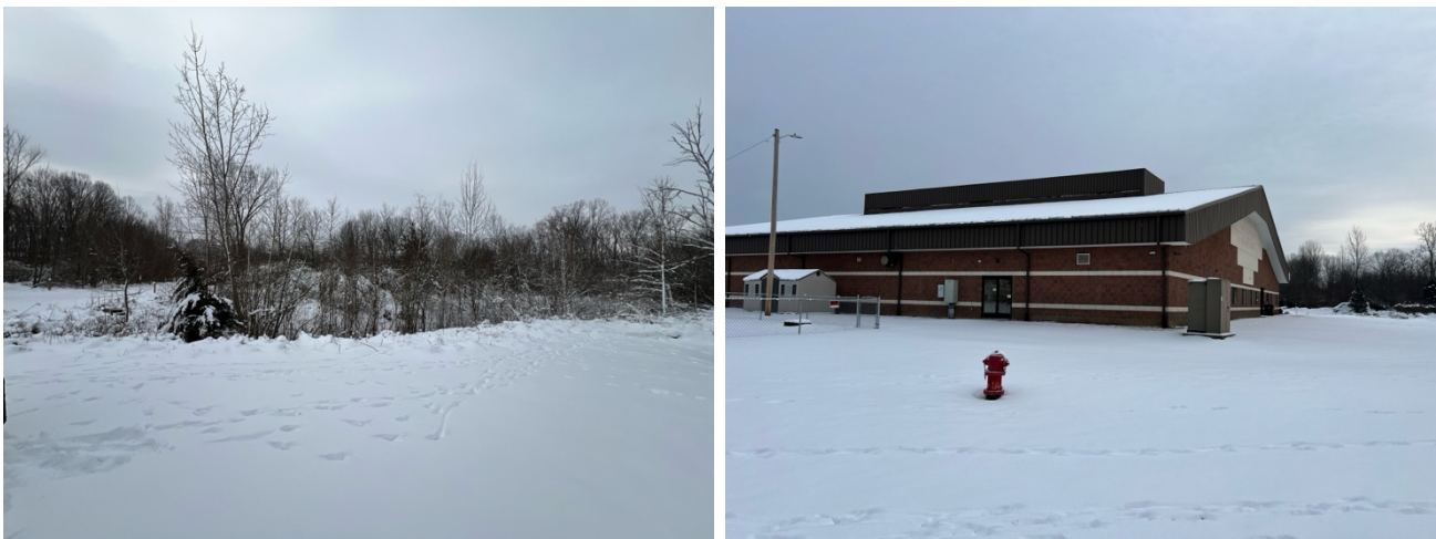
Figure 30. A) Parcel View and one of its wetlands. B) Existing Building on the site.
