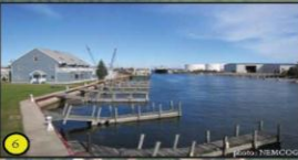
6 View of the US Coast Guard facility located just north of US Oil. Notice the easy access for docking of both large or small Coast Guard Cutters.
