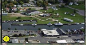
View looking east toward the Cheboygan Harbor Marina, which is located just north of East Park & presents pedestrian circulation opportunities.
