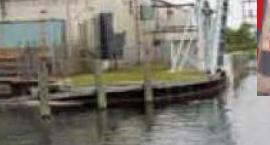
View looking south from the State St. bridge.
