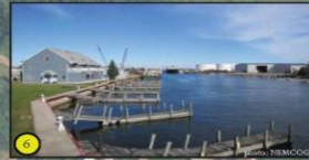
View of the US Coast Guard facility located just north of US Oil. Notice the easy access for docking of both large or small Coast Guard Cutters.
