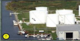
7 View of the US Oil bulk storage facility located just north of Walstrom Marine. Notice the easy access for docking and small amount of useable land currently available.
