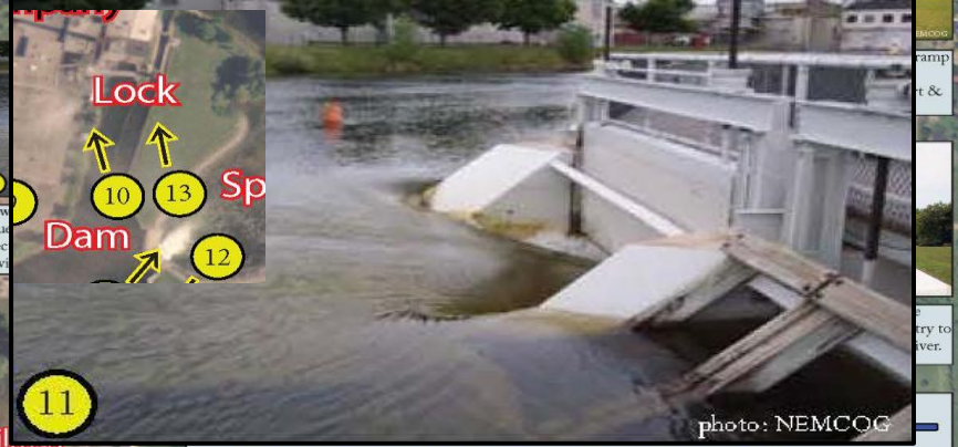
View looking south from the State St. bridge.
