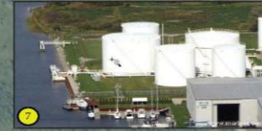
View of the US Oil bulk storage facility located just north of Walstrom Marine. Notice the easy access for docking and small amount of useable land currently available.
