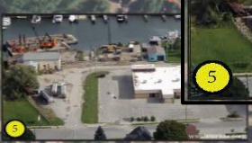
View of Ryba Marine Const. from above looking east towards the marina. Notice the close proximity of the working dock to the residential use to the south.
