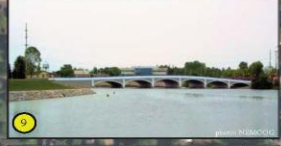
View looking south towards the Lincoln Avenue bridge. The stone seawall looks to be in good condition and fits in the surroundings very well.
