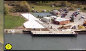
View of the US Coast Guard facility located just north of US Oil. Notice the easy access for docking of both large or small Coast Guard Cutters.
