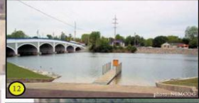
View looking west from the Lincoln Street Boat Access Site at two public boat ramps south of the dam and boat lock..
