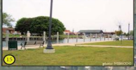
View looking northwest from the boat ramp area. Notice the pavement and site amenities present for pedestrian comfort & circulation.
