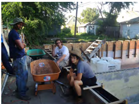
Waiting for cement truck
