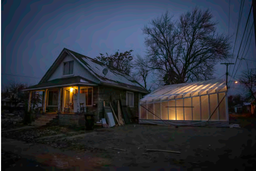
Afterhouse at completion of REI Part III funding – Fall 2014
