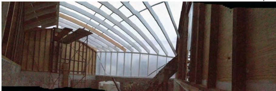
Interior view after REI Part III
