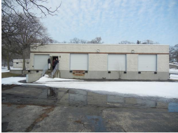
Rear loading dock
