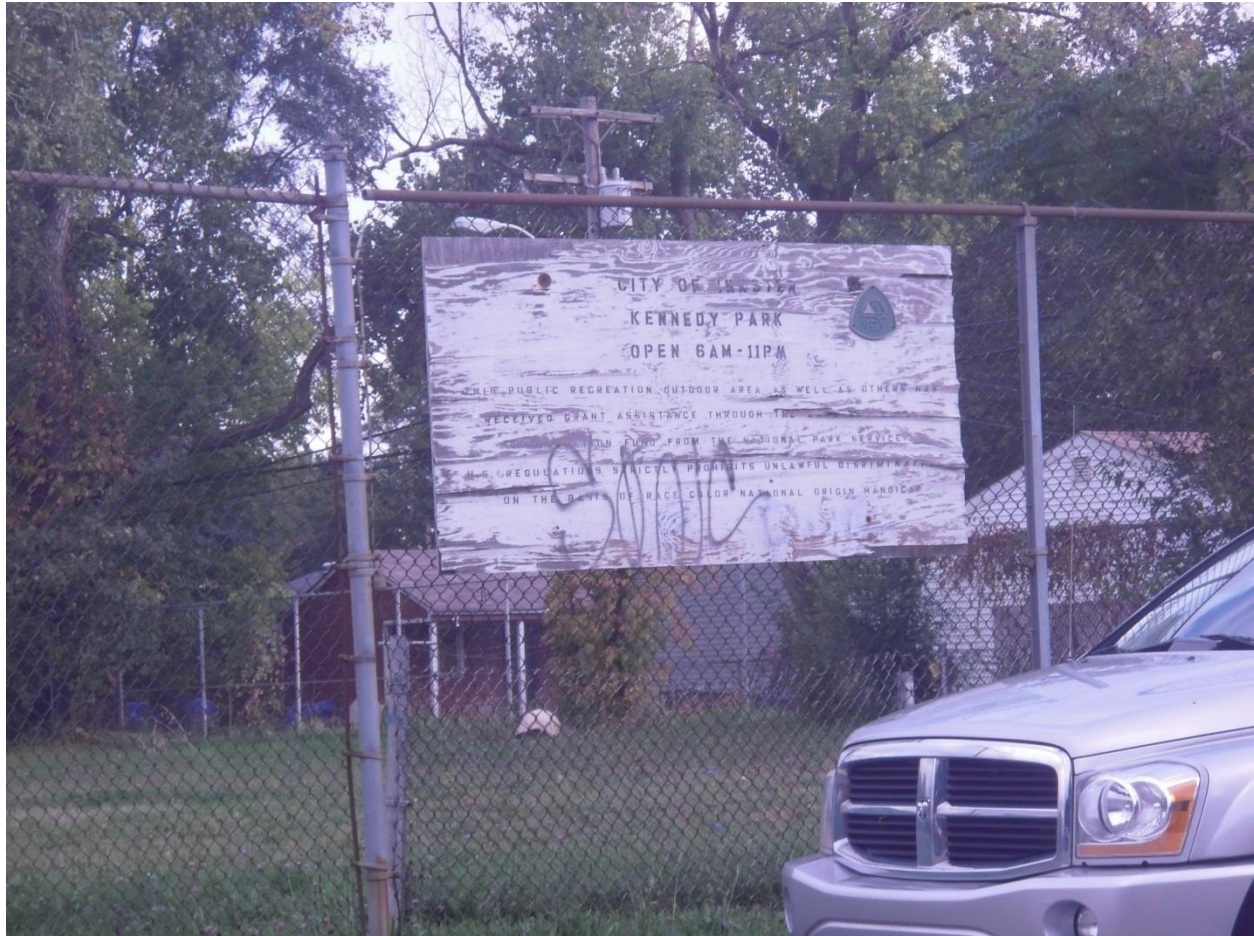
Figure 16. Disused ball diamond and vandalized, decrepit entry sign to Kennedy Park showing LWCF logo.
