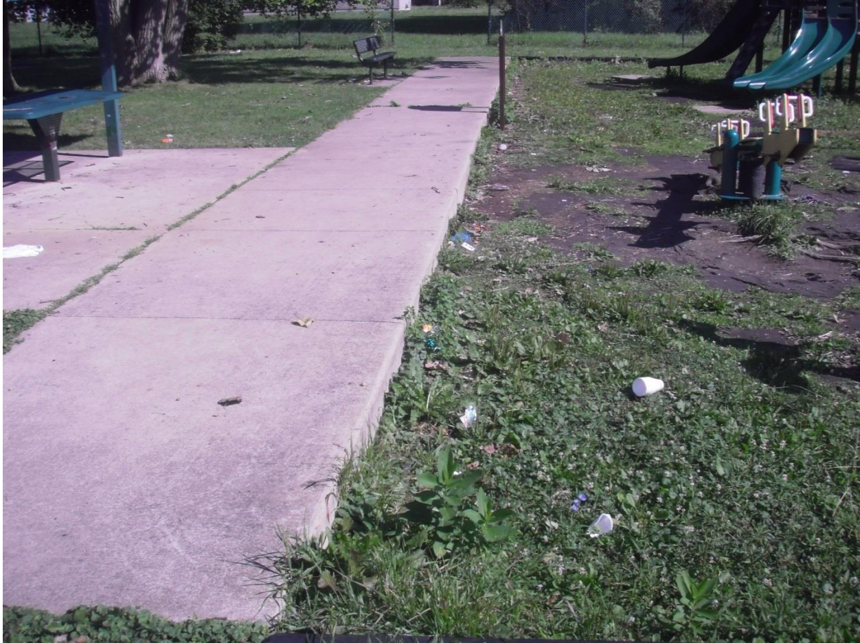
Figure 18. Inaccessible design for playground at Dartmouth with 4-6 inch dropoff to playground from sidewalk. In addition playground has litter, rolled filter fabric and lacks evidence of maintenance.
