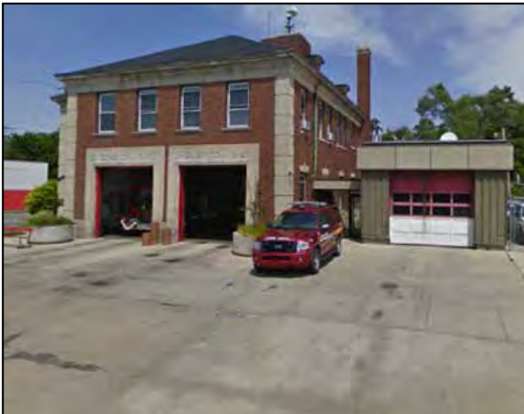
Figure 2.2: Detroit Fire Department Station on Joy Road.
