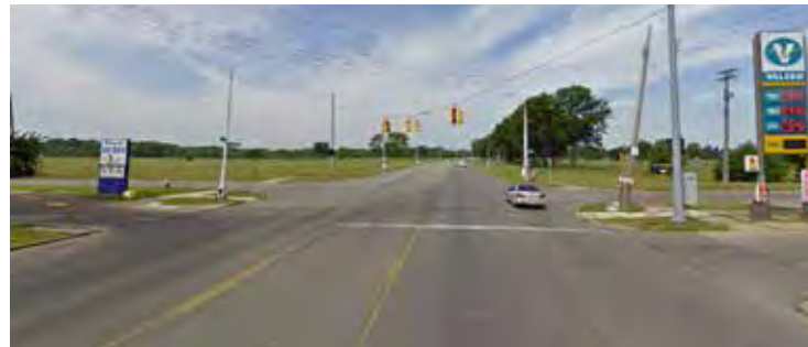
Figure 3.10: Joy Road and Trinity Road (Facing West)
