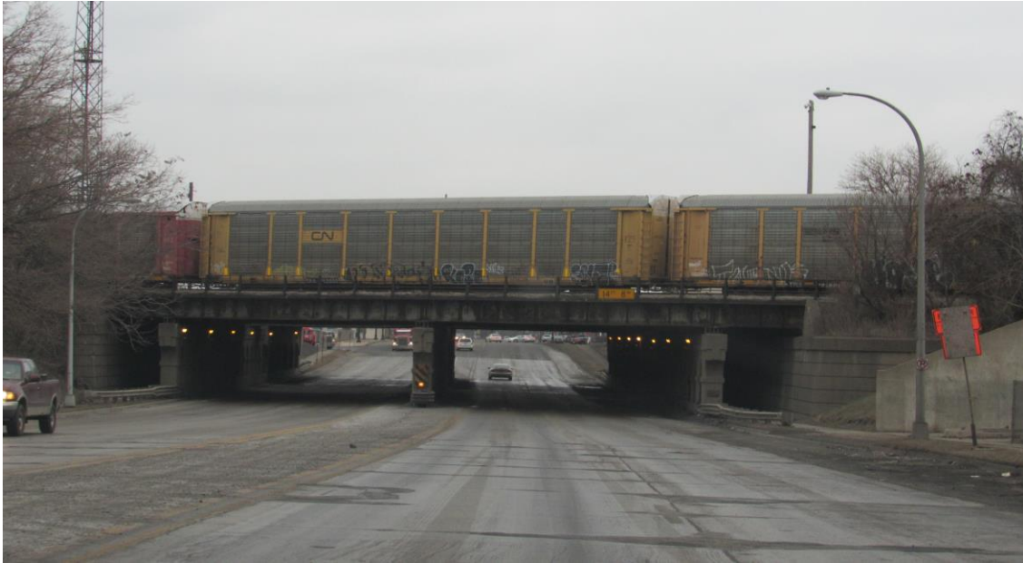
Figure 49: Dix-Vernor Corridor Viaduct
